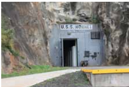
Waikele Storage Facilities
