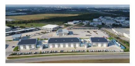
The 20.6-acre development consists of an Administration building, Crew building, Utility building, Warehouse, Material Storage and Laydown Yard, a Wash Bay, a large surface parking area for City fleet vehicle and equipment parking, and an ~500KW photovoltaic system. In addition to the solar array, there are four 18,000-gallon rainwater capture cisterns, high recycled content building materials, low-flow plumbing fixtures, and drought-tolerant plants and grasses.
